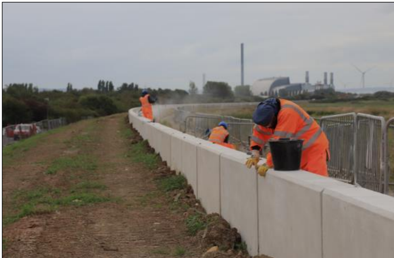
Plate A.2 Precast concrete flood wall 7
